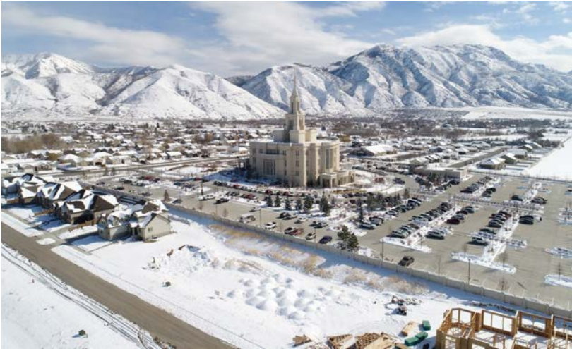
Figure 1-1: New Construction around LDS Temple.
