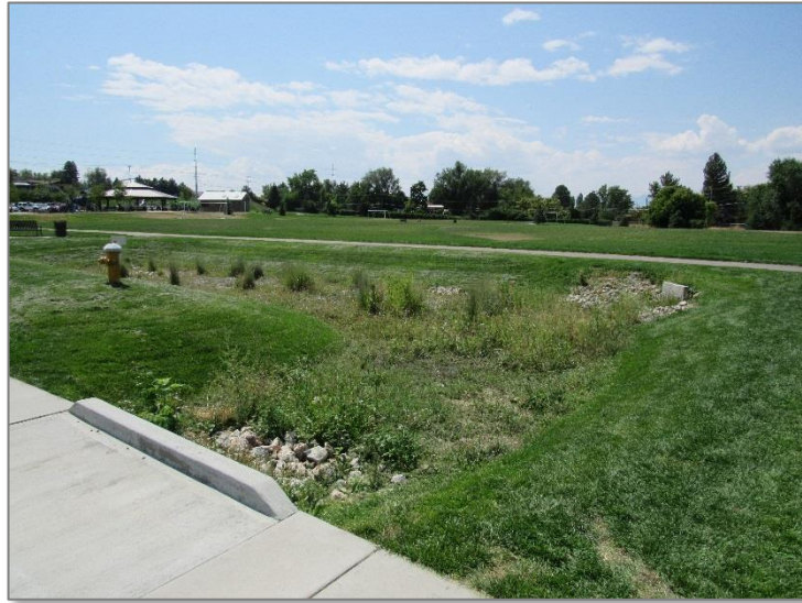
Figure 14: Bioretention area at Mountview Park.
