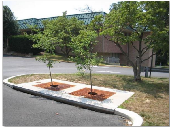
Figure 20: Proprietary tree box filter.
