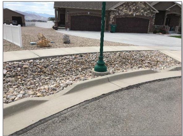
Figure 9: Curb cuts to a rock lined swale.
