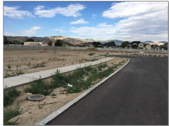
Figure 18: A vegetated swale that will provide pretreatment for a dry well.
