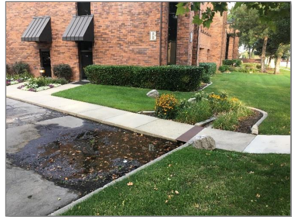
Figure 17: Standing water after a rain event at a bioretention BMP.
