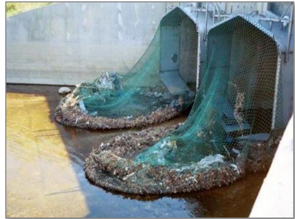
Figure 5: End-of-pipe trash netting.
