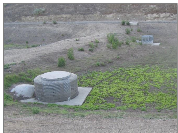
Figure 4: Multi-stage overflow outlet with trash screen.
