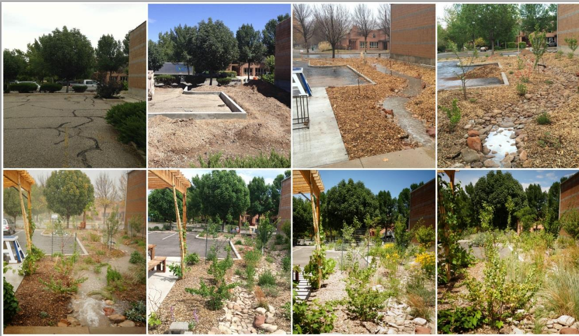
Figure 16: Construction progress of permaculture garden.
