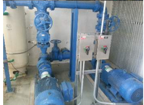
Figure 3-15 DAF Air Panel
