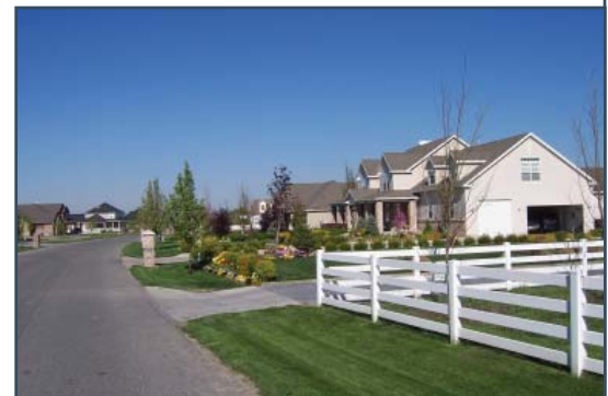
An example of a drainage swale or ditch that is to be included in rural density road cross-sections. The manicured landscaping shown in this image is not appropriate for rural density developments.
