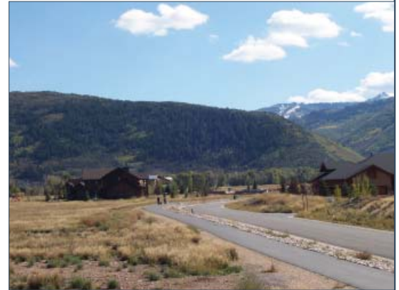
Class I trails may be paved and adjacent to a roadway, but separated by a small median.
