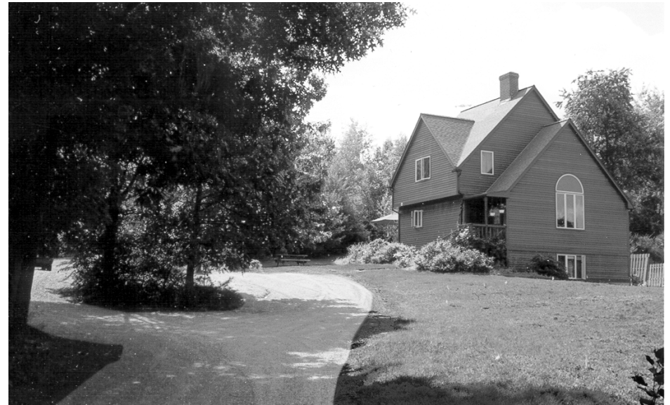
Gravel driveways are characteristic of the surrounding rural area and did not detract from the aesthetics of the development or the affordable housing (single family affordable unit shown here).
