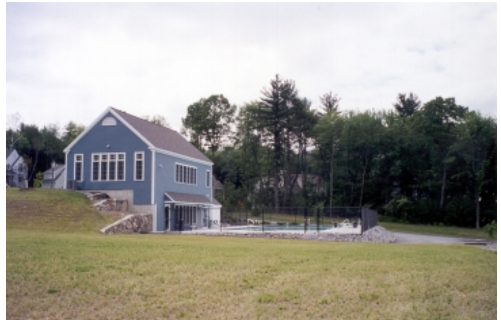
The central community open space area consists of a club house, in-ground pool (on right), tennis courts (on left) and an open field as seen in the foreground.
