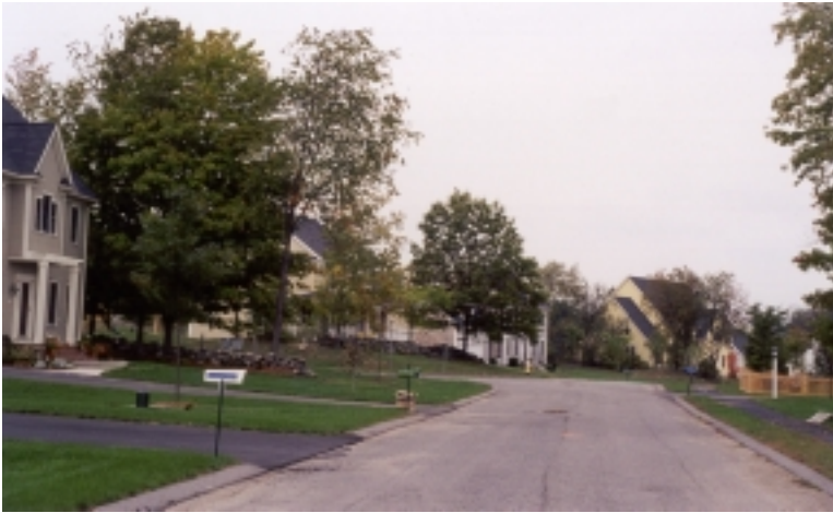
Roads are 24' wide; granite curbing was unnecessary and therefore not required. Several stone walls were preserved by this design. At the time this report was written, the developers' obligations to the roadways were not yet completed.
