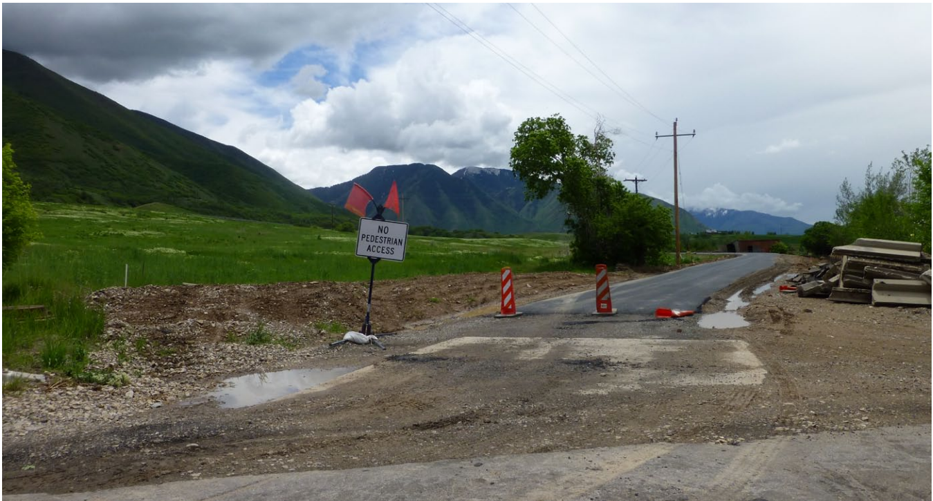
Construction of the Mapleton Parkway Trail, May 2016
