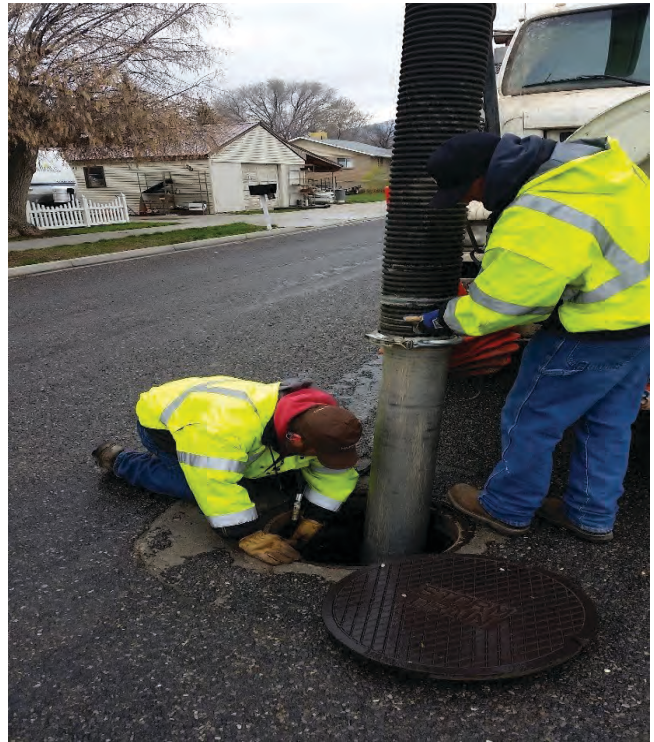
Source: Payson. Payson sewer construction. April, 2016. Facebook.com.
